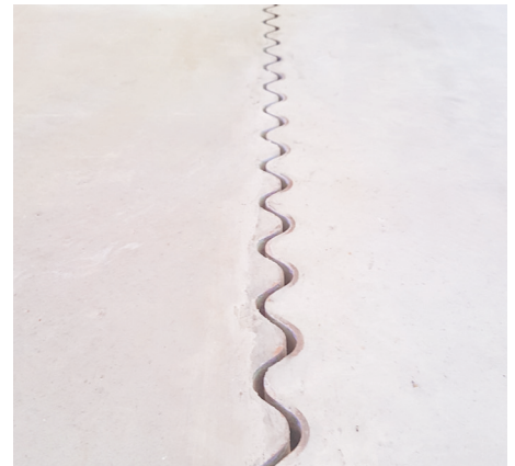
Co-sinus steel armoured construction joint - providing smooth load transfer trafficked areas for high MHE.
