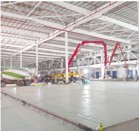
Preparation is one of many critical success factors. Slip membrane laid in preparation for next concrete pour.
