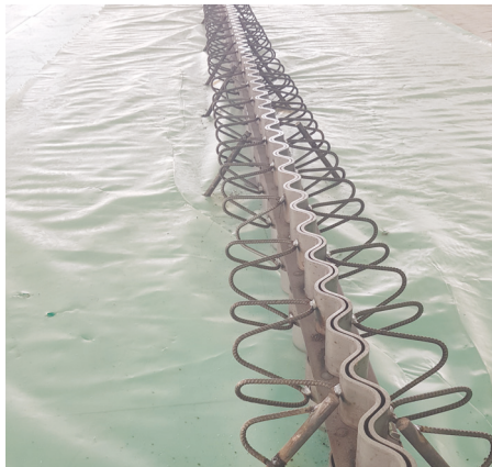
Co-sinus steel armoured construction joint - providing smooth load transfer trafficked areas for high MHE.
